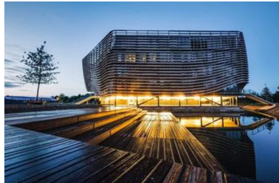
Figure 1. Wetsus building in Leeuwarden (NL).
