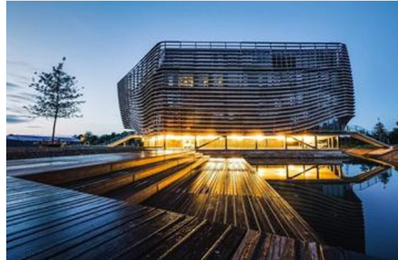
Figure 1. Wetsus building in Leeuwarden (NL).
